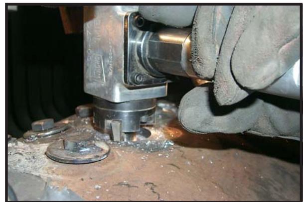
MB Beveler machining Header using special “Stub Tube” removal tool bit.
