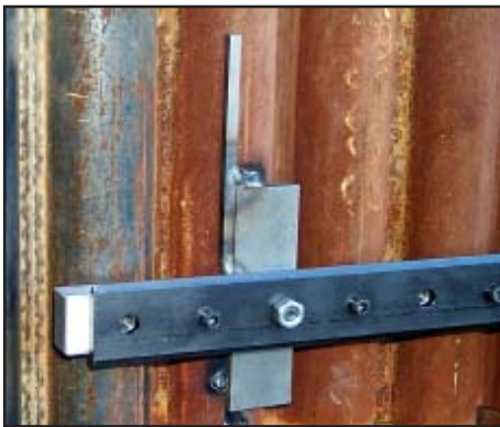
Weld tab and track assembly
